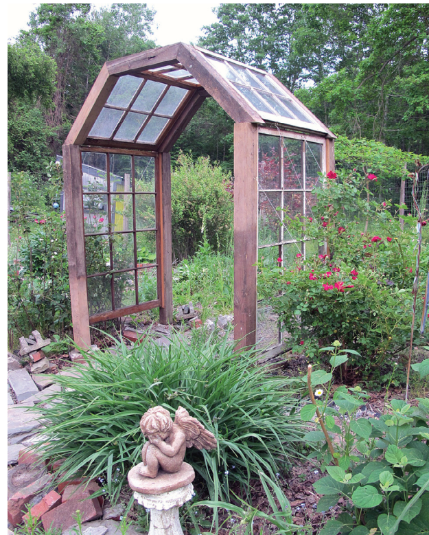
Trellis made from reclaimed old wooden framed windows.
